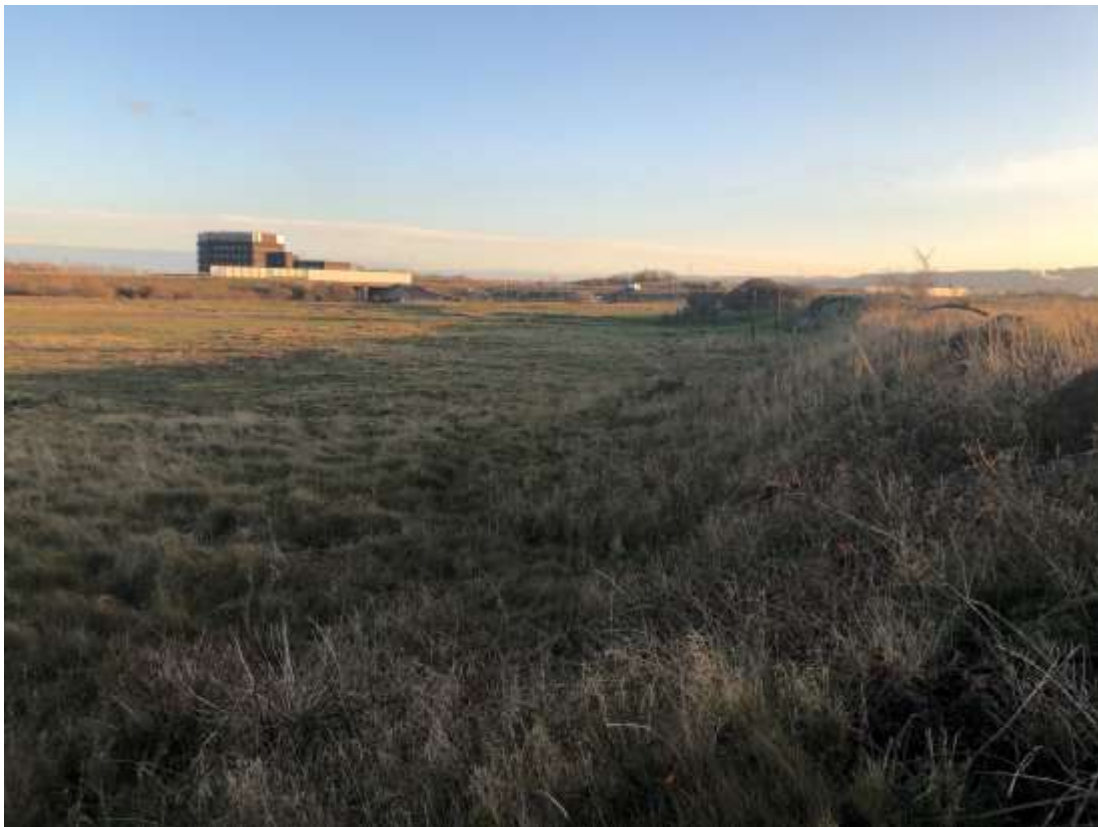
Plate 2: View from ground level in Long Acres. The road can be seen raised up on an embankment in front of the Steel House
